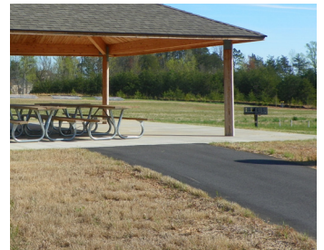
ADA Trail Access to Shelter and Restroom
